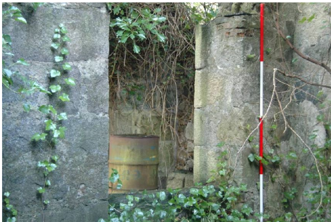
Illus 119 Building 24, detail of window molding.
