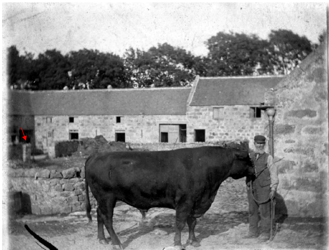
Illus 120 Photograph of the steading E court showing enclosed central yard. Man with bull standing by W gable of building 3. Mill building 7 in RHS background, with Buildings 10, 11 to LHS. The archway into the courtyard (red arrow) can just be seen in LHS. Note the tall stable doors and slit ventilators of the W wall of Building 10. (Blairs Museum T1001-8)
