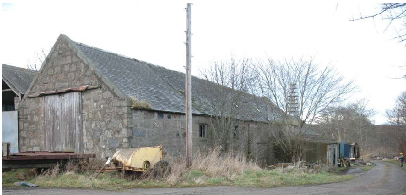
Illus 114 Building 7: The Mill, looking NNE. The wheel would have been near the position of the small tree behind the GPO pole.
