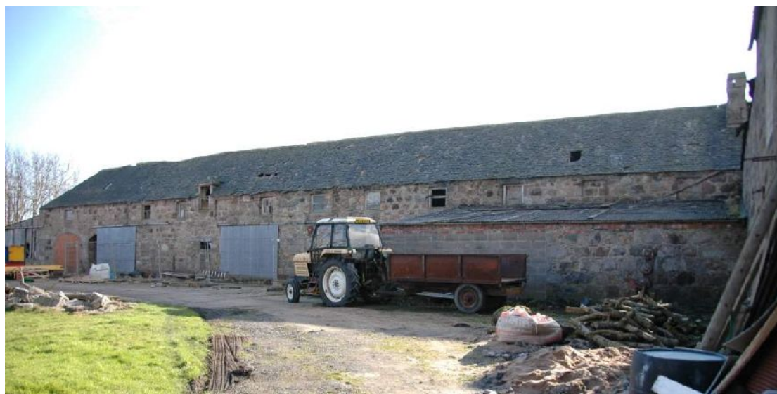
Illus 116 Looking SE across the frontage of Buildings 13 and 10. Note the arches at far end (Building 10). The LHS arch was carriage bay. Next to it, partially covered by metal door is archway into central courtyard.
