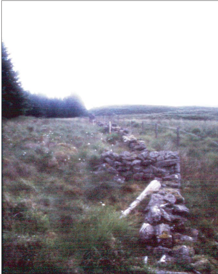
Plate 1. General view of the dyke facing North West
