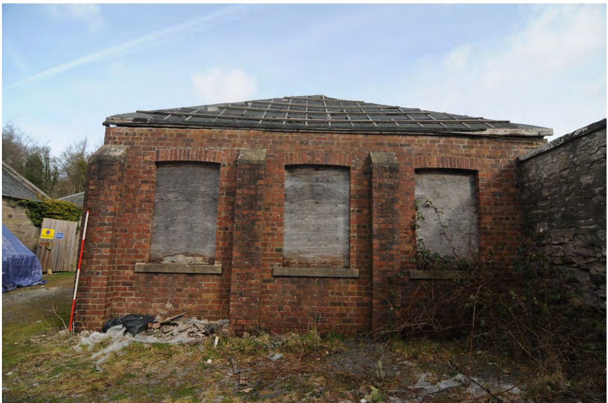
Fig 20: Phase 5, Garage, Unit 6, external south-facing elevation
