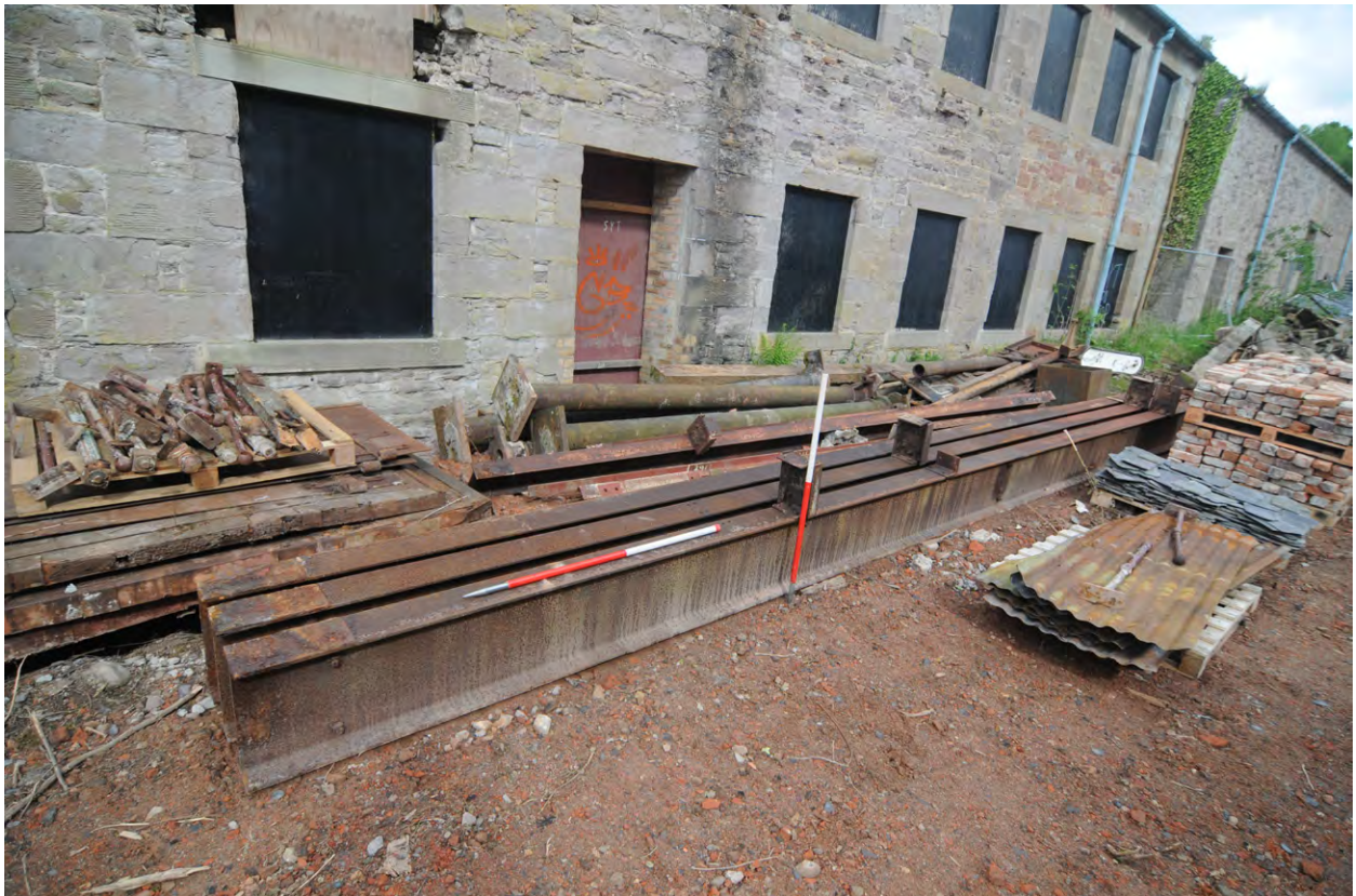
Fig 30: I beams salvaged from demolition
