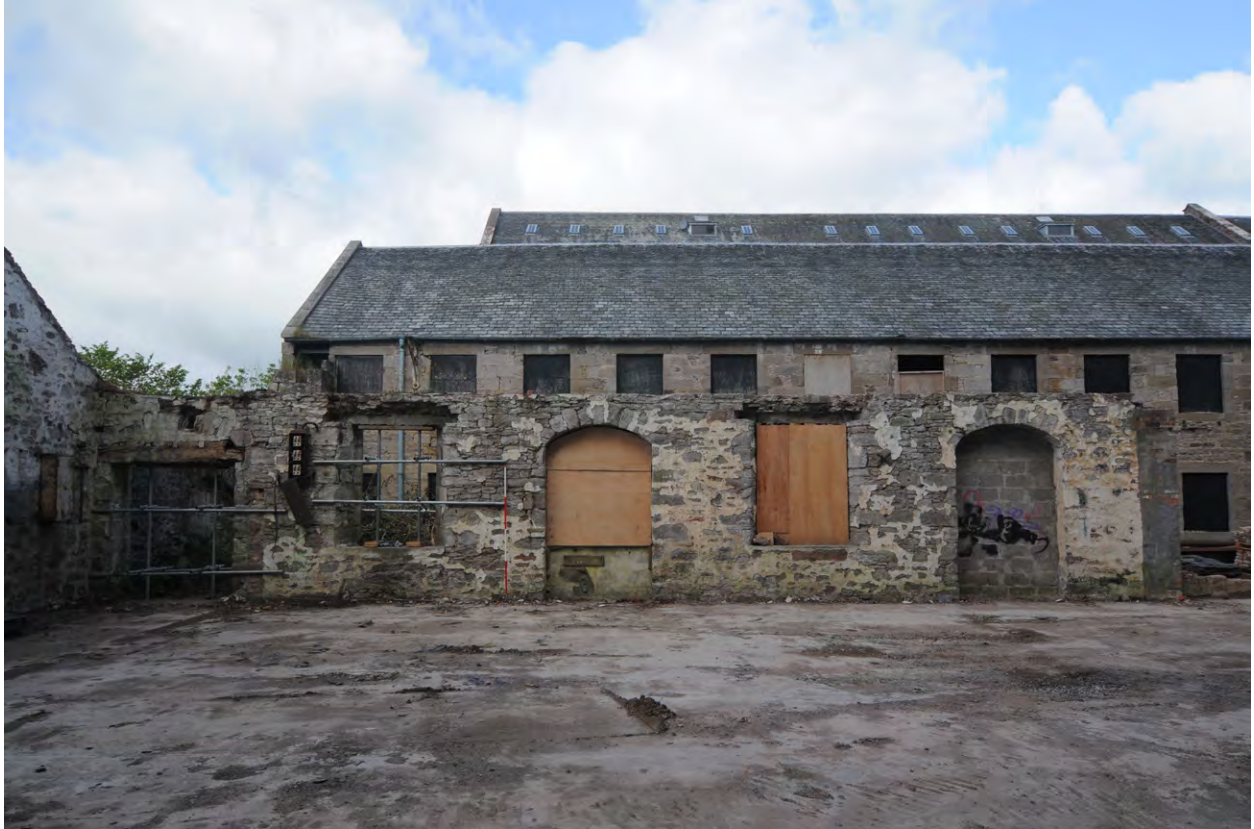
Fig 9: Phase 1, internal east-facing elevation of Unit 2
