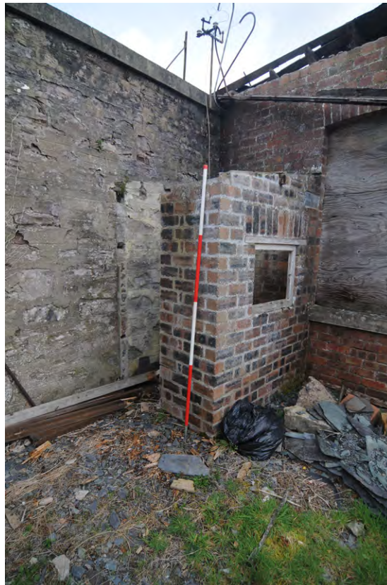
Fig 24: Phase 5 toilet, Unit 7 next to Garage
