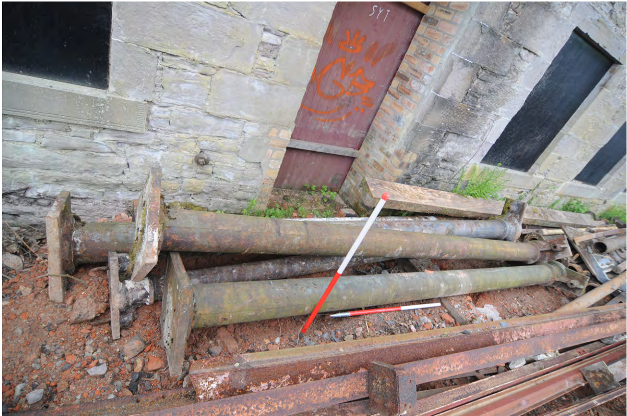
Fig 31: The Phase 1 cast columns salvaged from the demolition of Unit 2
