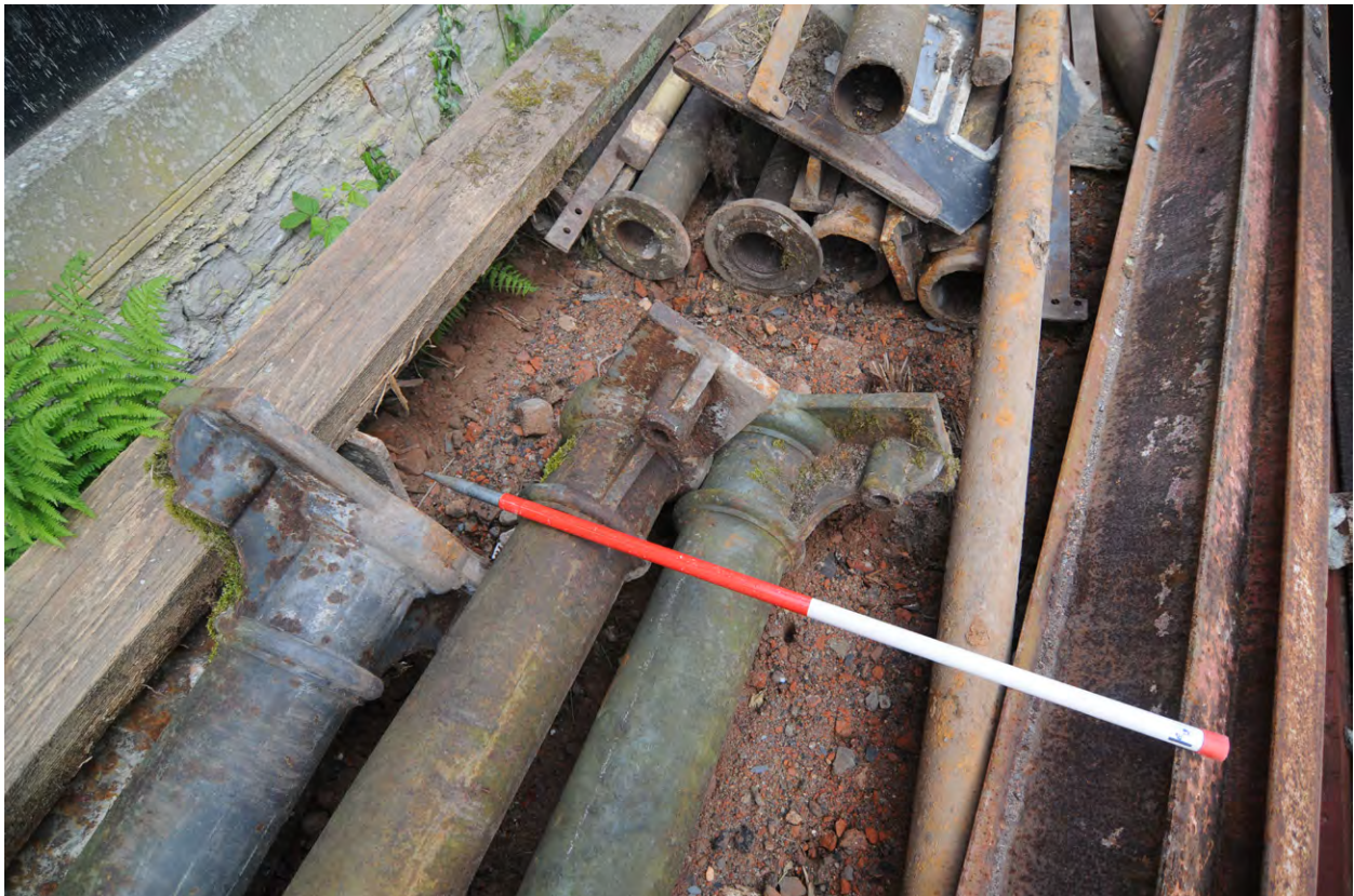
Fig 32: Detail of the heads of the Phase 1 cast columns salvaged from the demolition of Unit 2
