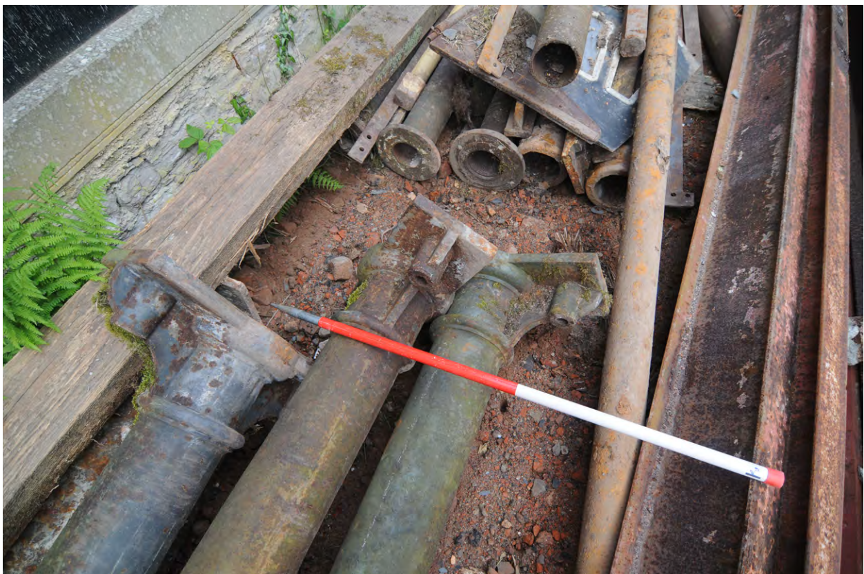
Fig 32: Detail of the heads of the Phase 1 cast columns salvaged from the demolition of Unit 2
