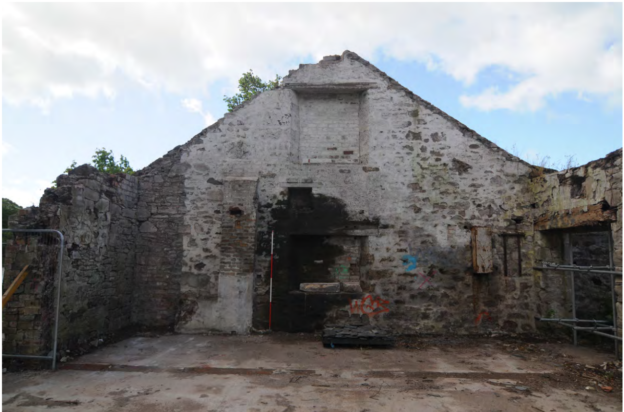
Fig 8: Phase 1, internal north-facing elevation of Unit 1
