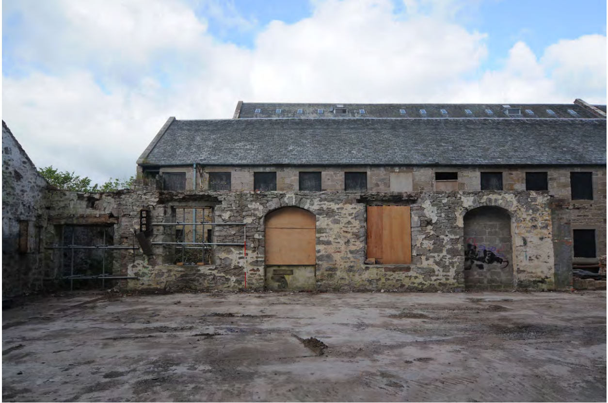
Fig 9: Phase 1, internal east-facing elevation of Unit 2
