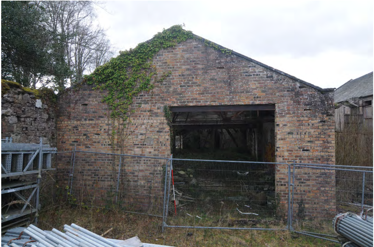
Fig 26: Phase 6 external north-facing elevation, Unit 4, showing doorway (027)
