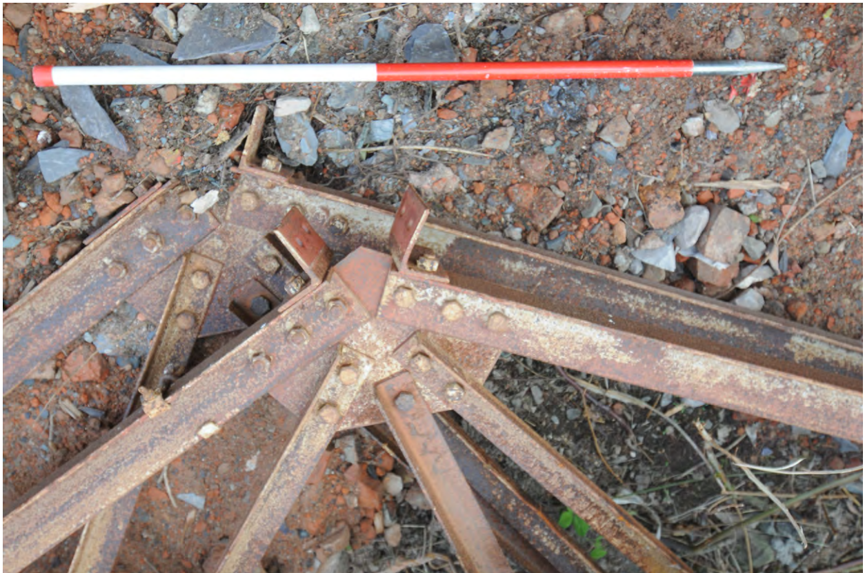
Fig 34: Detail of the Phase 1 metal roof trusses salvaged from the demolition of Unit 2 showing where they would have bolted onto a ridge beam
