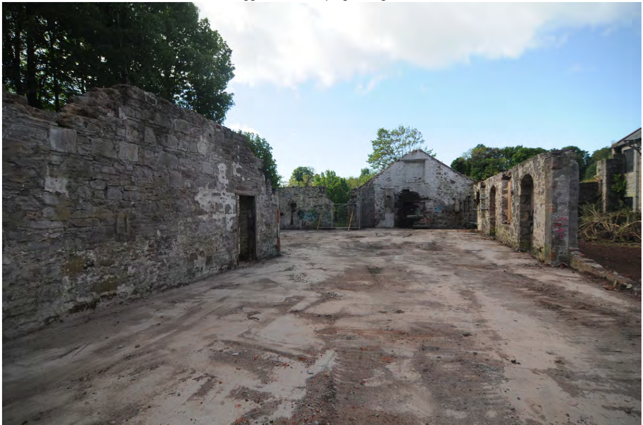
Fig 28: Site post partial demolition
