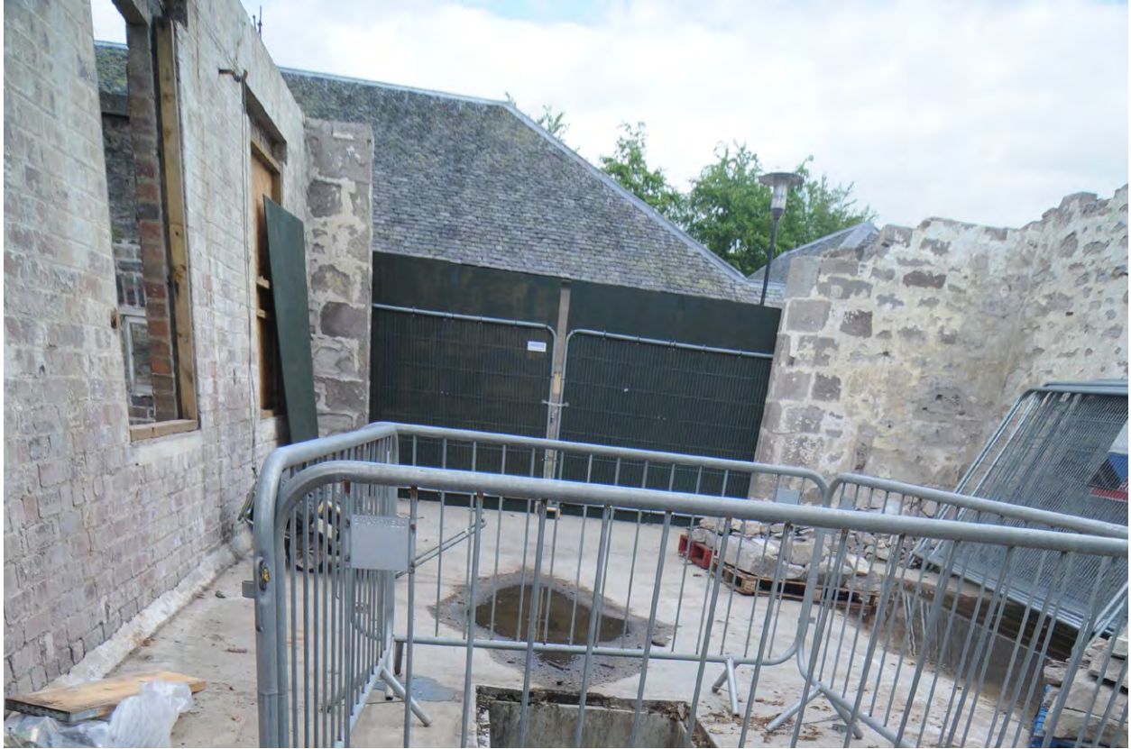
Fig 23: Phase 5, Garage, Unit 6, vehicle inspection pit
