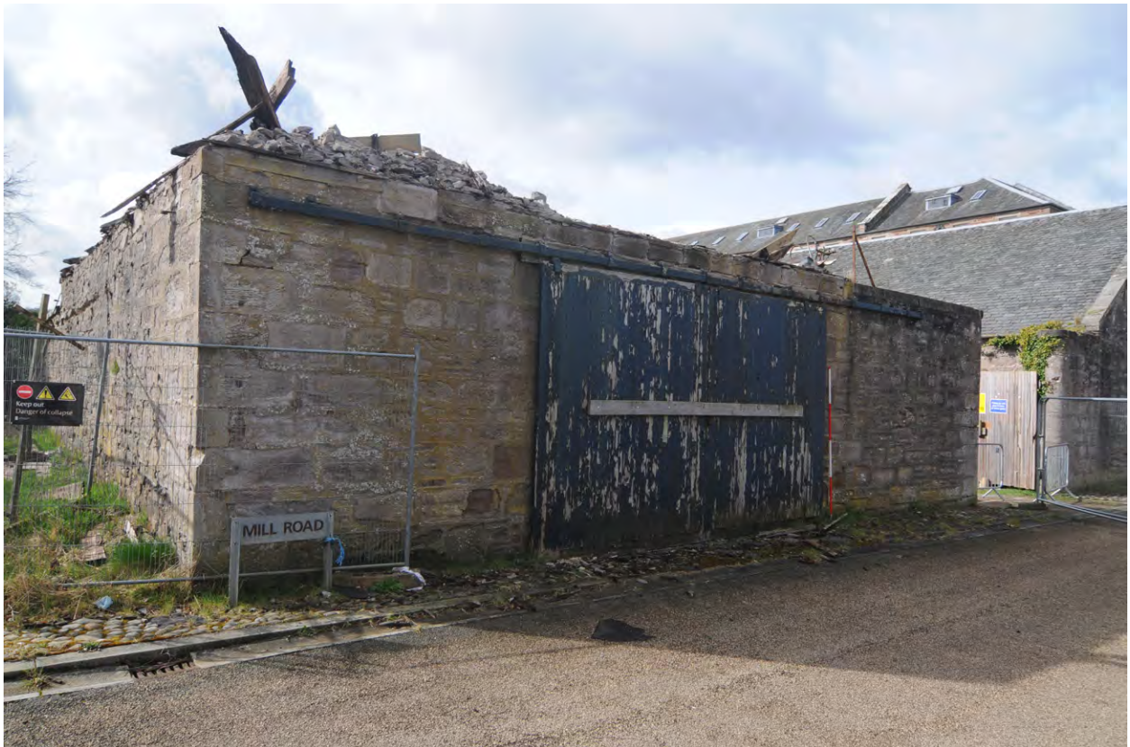
Fig 22: Phase 5, Garage, Unit 6, external north-facing elevation with double door (072)
