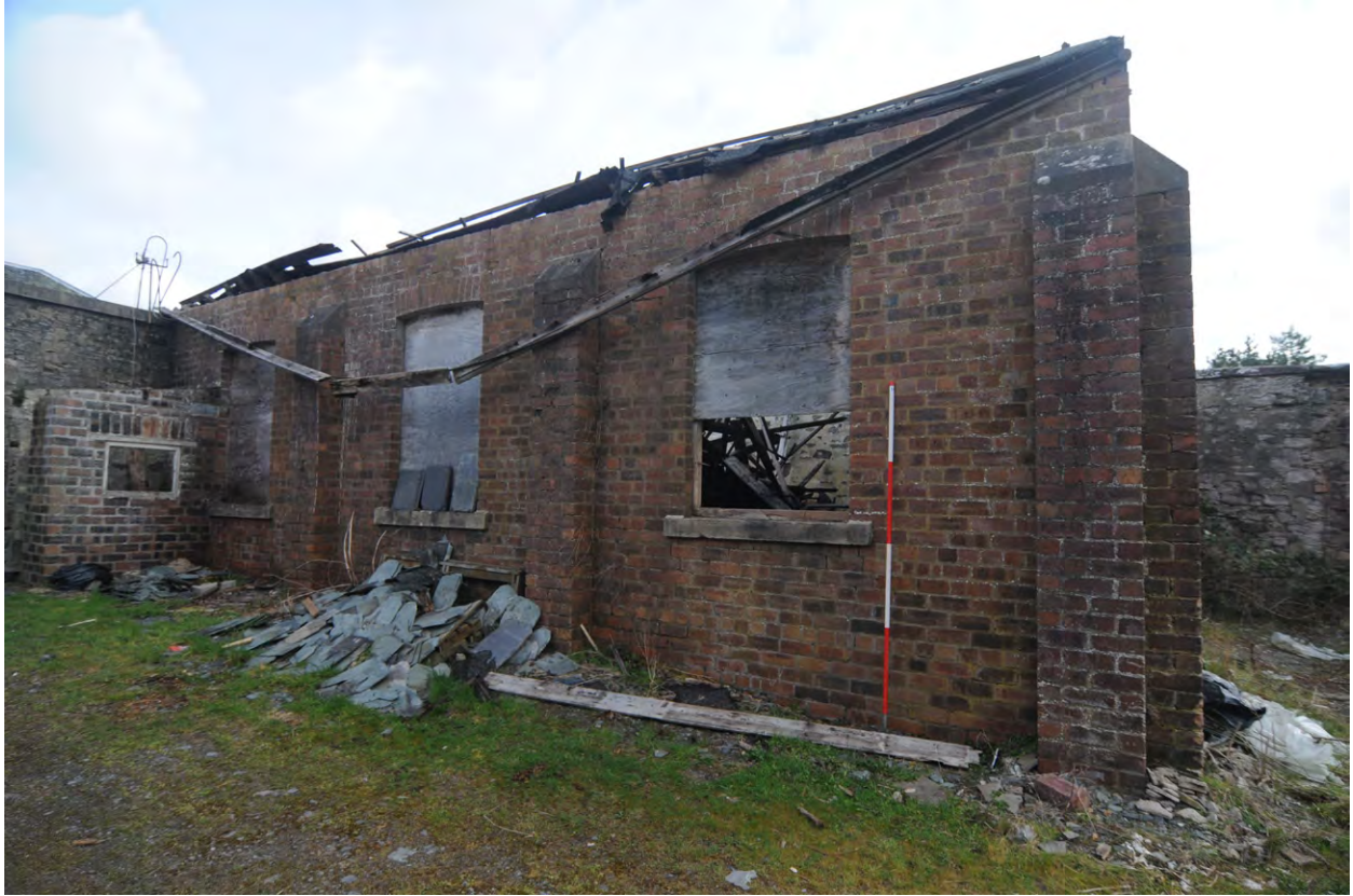
Fig 21: Phase 5, Garage, Unit 6, external west-facing elevation
