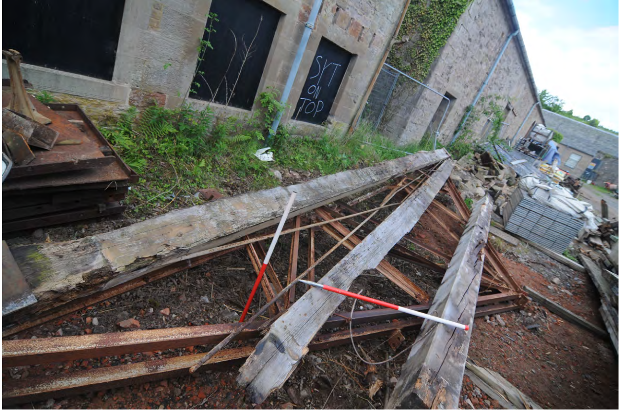
Fig 33: The Phase 1 metal roof trusses salvaged from the demolition of Unit 2
