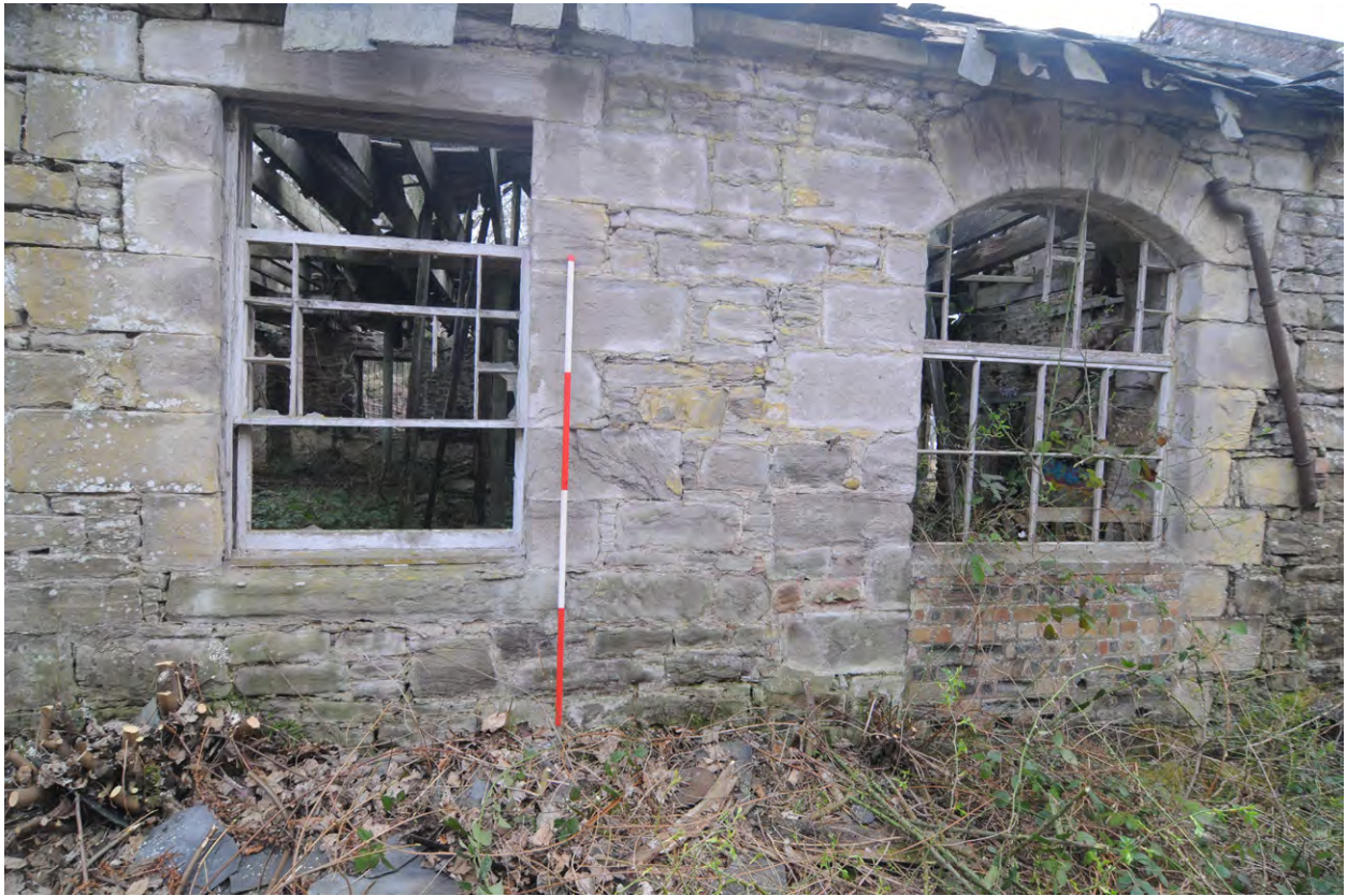
Fig 7: Phase 1, blocked doorway (031) and window (033)
