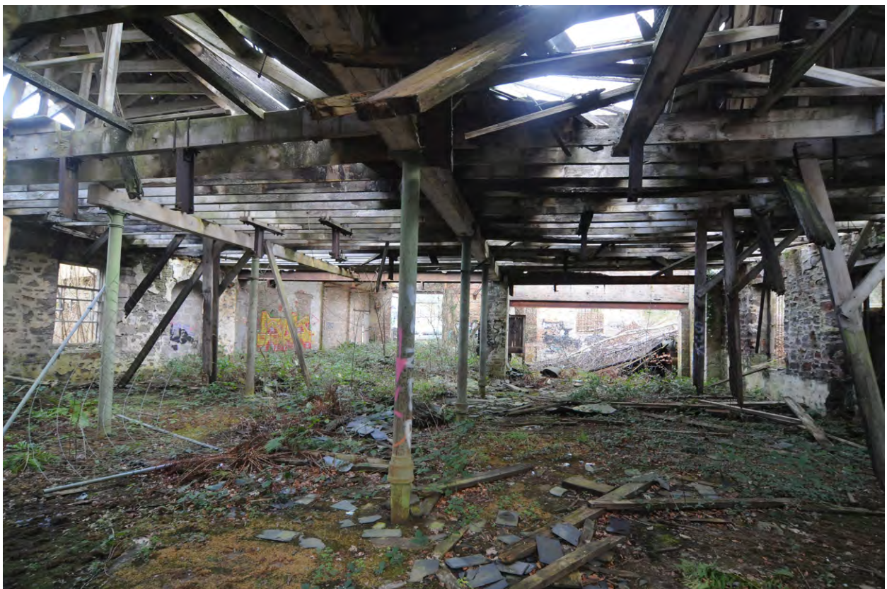
Fig 12: Phase 3 line of internal columns supporting roof when Phase 3 removed eastern wall of Unit 2
