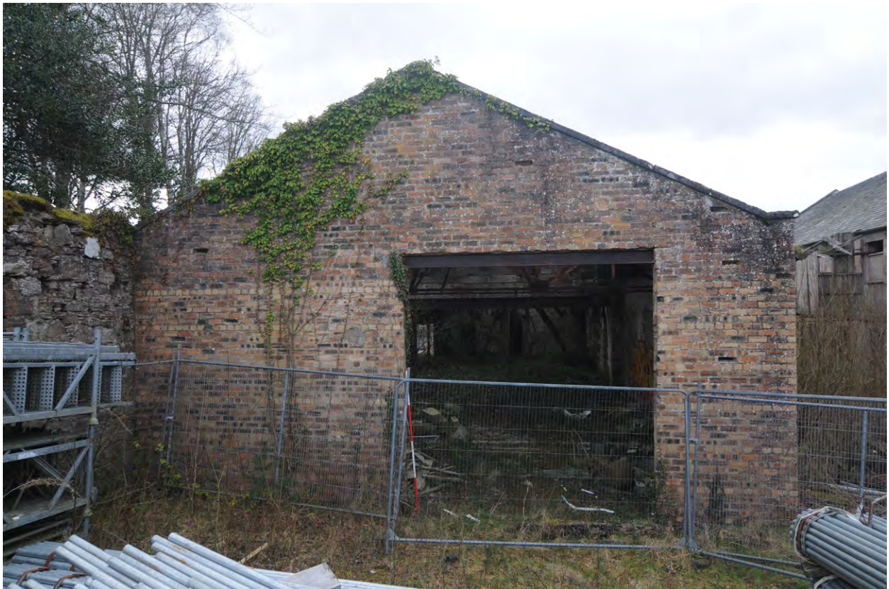
Fig 26: Phase 6 external north-facing elevation, Unit 4, showing doorway (027)
