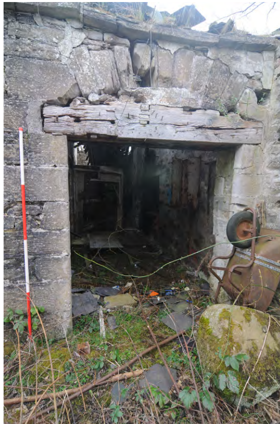
Fig 6: Phase 1, detail of reused lintel on doorway (029)
