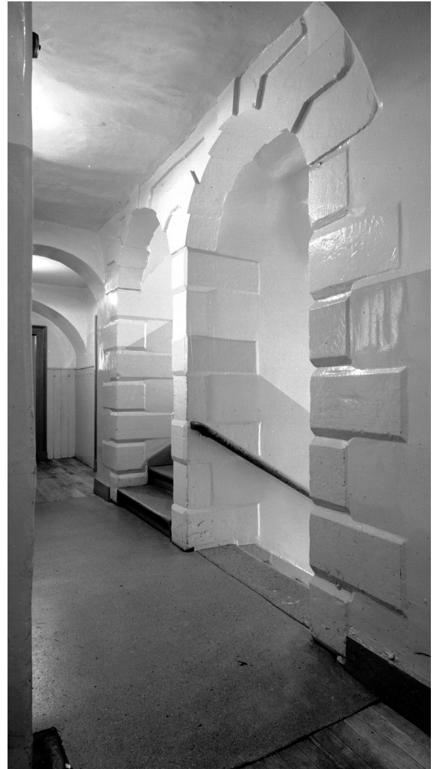
FIGURE 12 1998 view of arch staircase surround on second floor of 'Auld House'.
