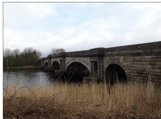
Plate 1: General shot of the bridge from the south side.
