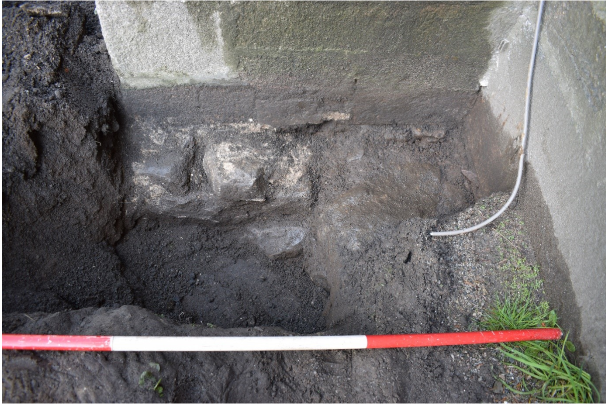
Illus 18 TP11 showing mortar bonded buttress foundation F1 (left) and wall foundation F2 (right); facing N
