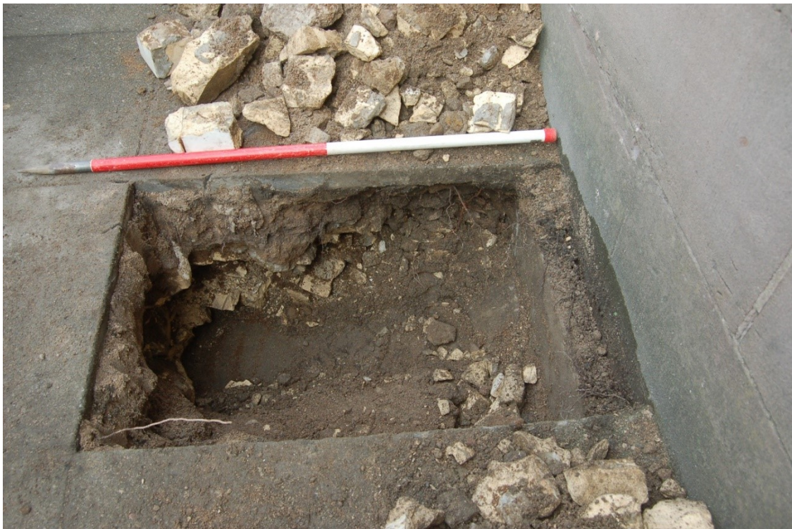
Illus 9 Dark grey cement surface visible beneath rubble fill of Test Pit 3: facing N.
