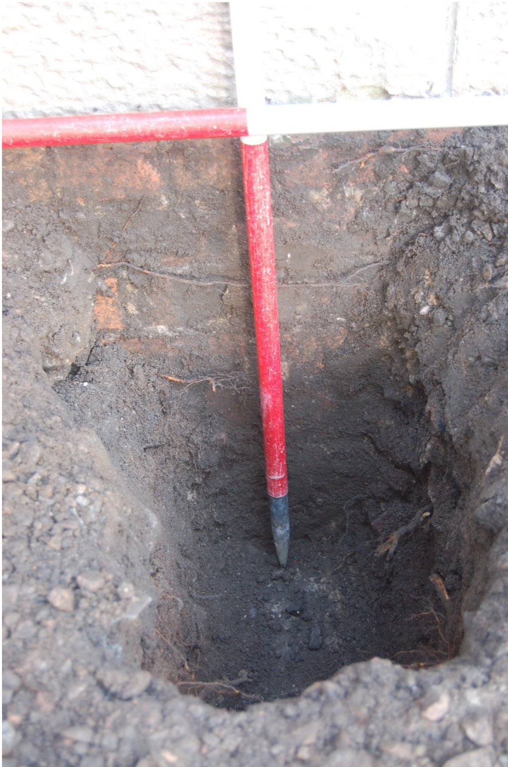
Illus 4 S facing exposed wall showing stone above bricks on a concrete foundation in Test Pit 1: facing N.
