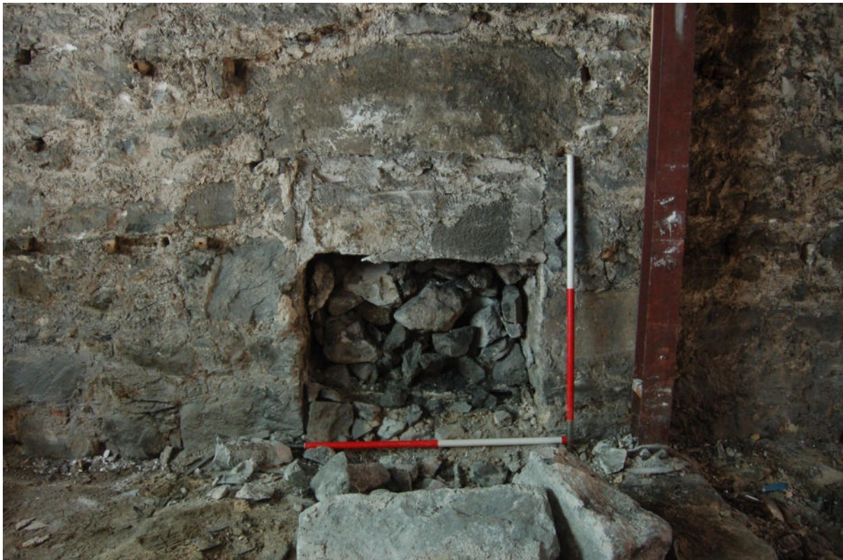
Illus 3 N- most hearth infilled with stone rubble within the ESE wall; facing ESE.
