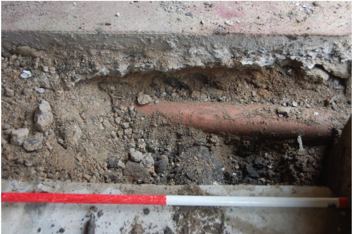
Illus 9 Section of drain located within Trench 1; facing E.
