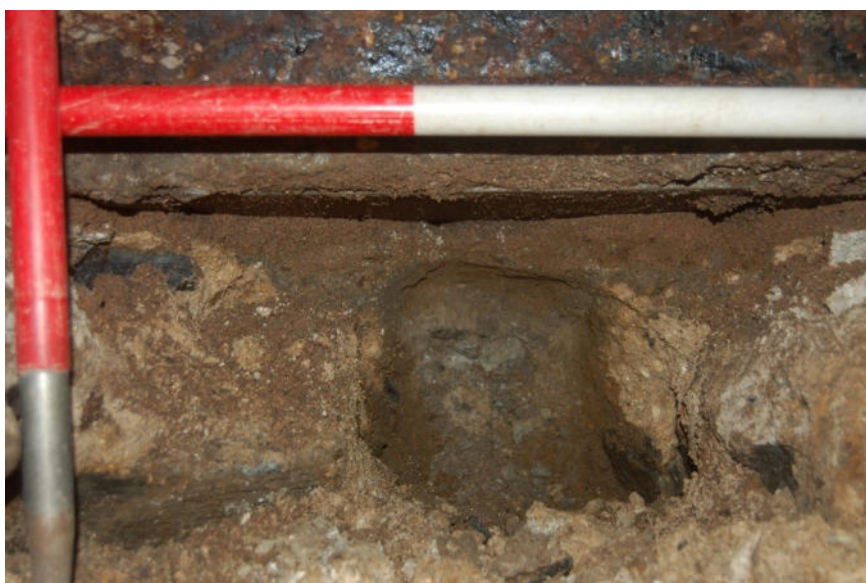
Illus 16 Rear face of cut granite stones facing the N wall of the building revealed by removal of a rough foundation stone from beneath the I-beam; facing N.
