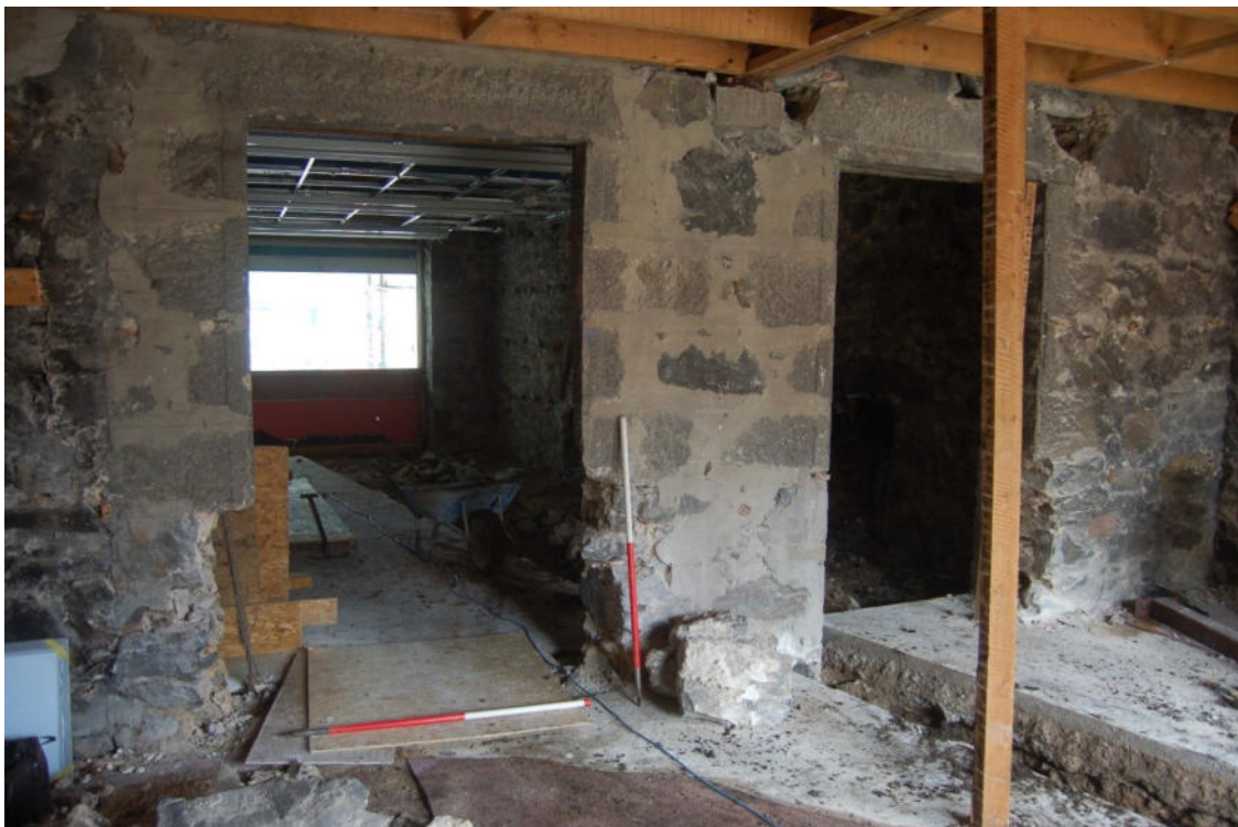
Illus 6 Window (L) and doorway (R) with ashlar dressed surrounds in the rear wall of the earlier building; facing NE.
