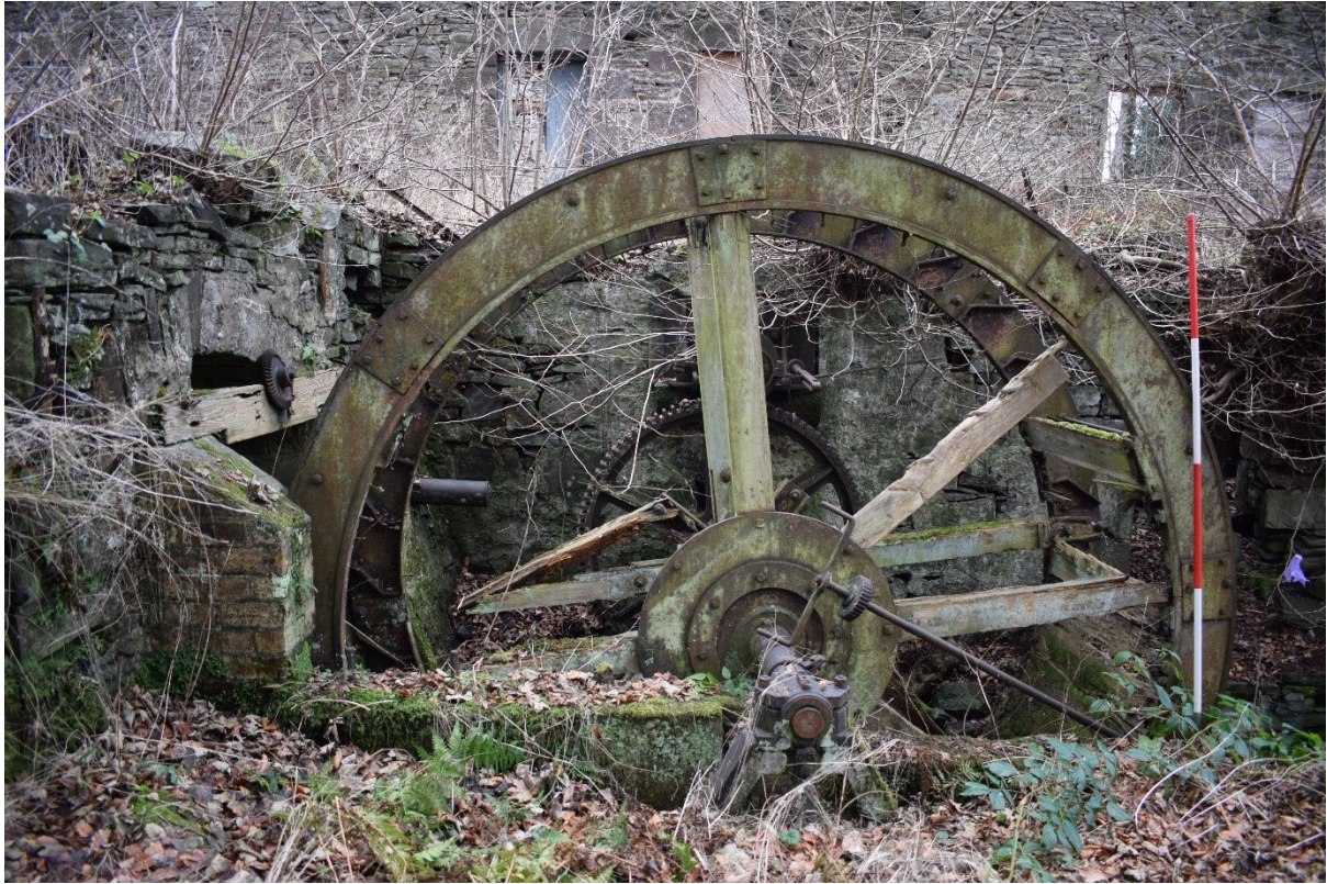
Illus 15 Mill wheel F17 in wheel pit Room 6; facing NNW
