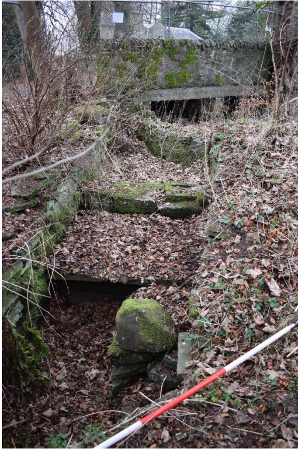
Illus 17 Lade F21 with bridge F19 (top) divided into lade to wheel (right) and overflow lade (left); facing NW
