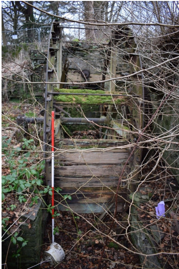
Illus 16 Mill wheel F17 in wheel pit Room 6; facing WSW
