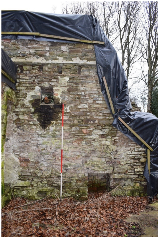
Illus 22 Room 3 NNW wall with wheel mechanism drive shaft F6 (top left) and aperture F7 (bottom right); facing NNW
