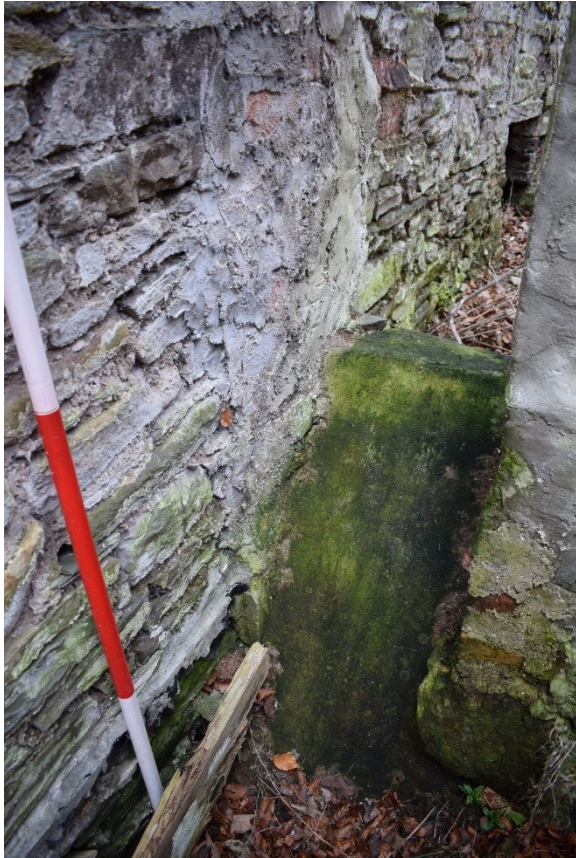
Illus 13 Concrete wheel-pit ENE of F4 within F1; facing NE
