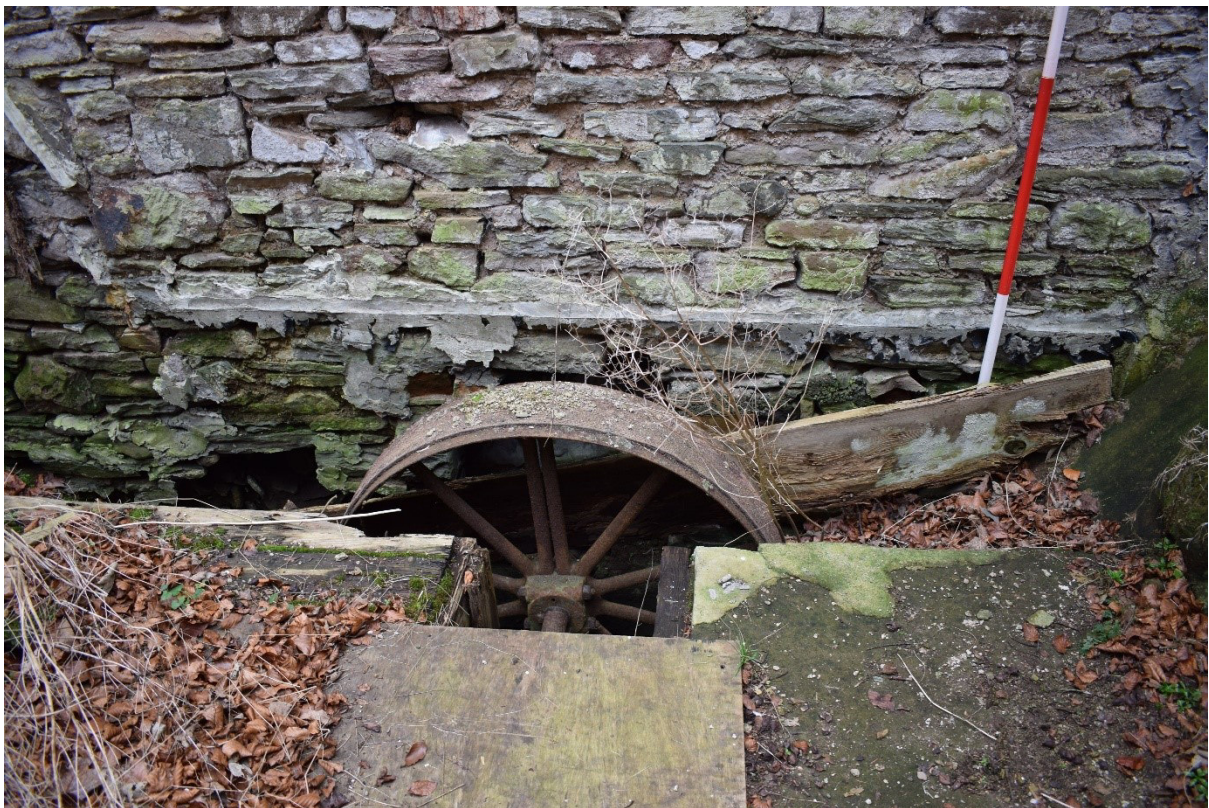
Illus 12 Room 1 wheel F4 in wheel-pit F2; facing NNW
