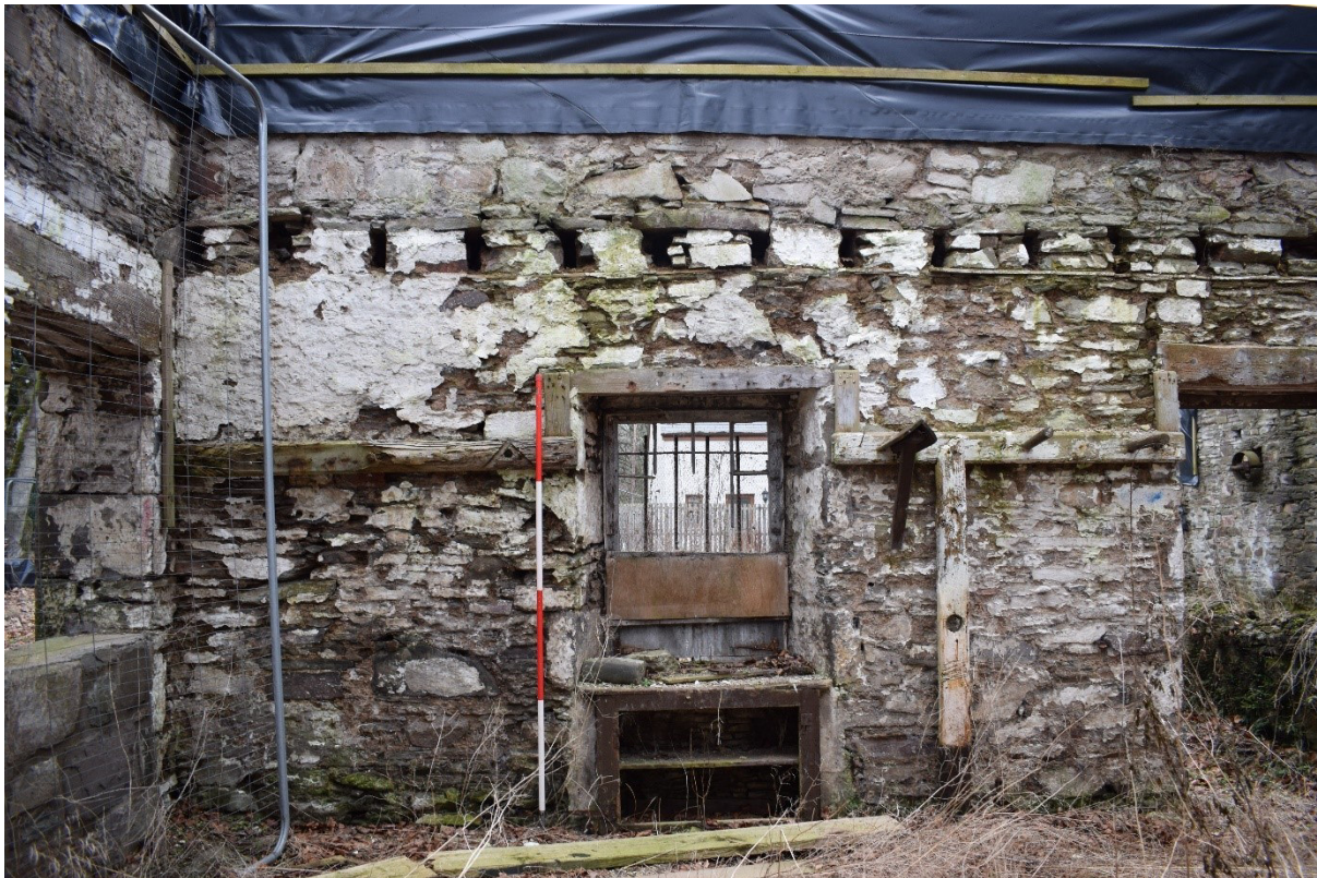
Illus 25 ENE wall Room 2 with W9 (centre) with cupboard in situ below and wooden saddle and harness storage F10 (right); facing ENE
