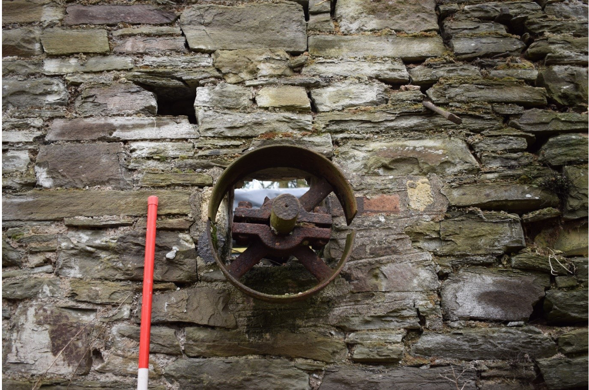
Illus 23 F6 wheel mechanism NNW side of wall; facing SSE
