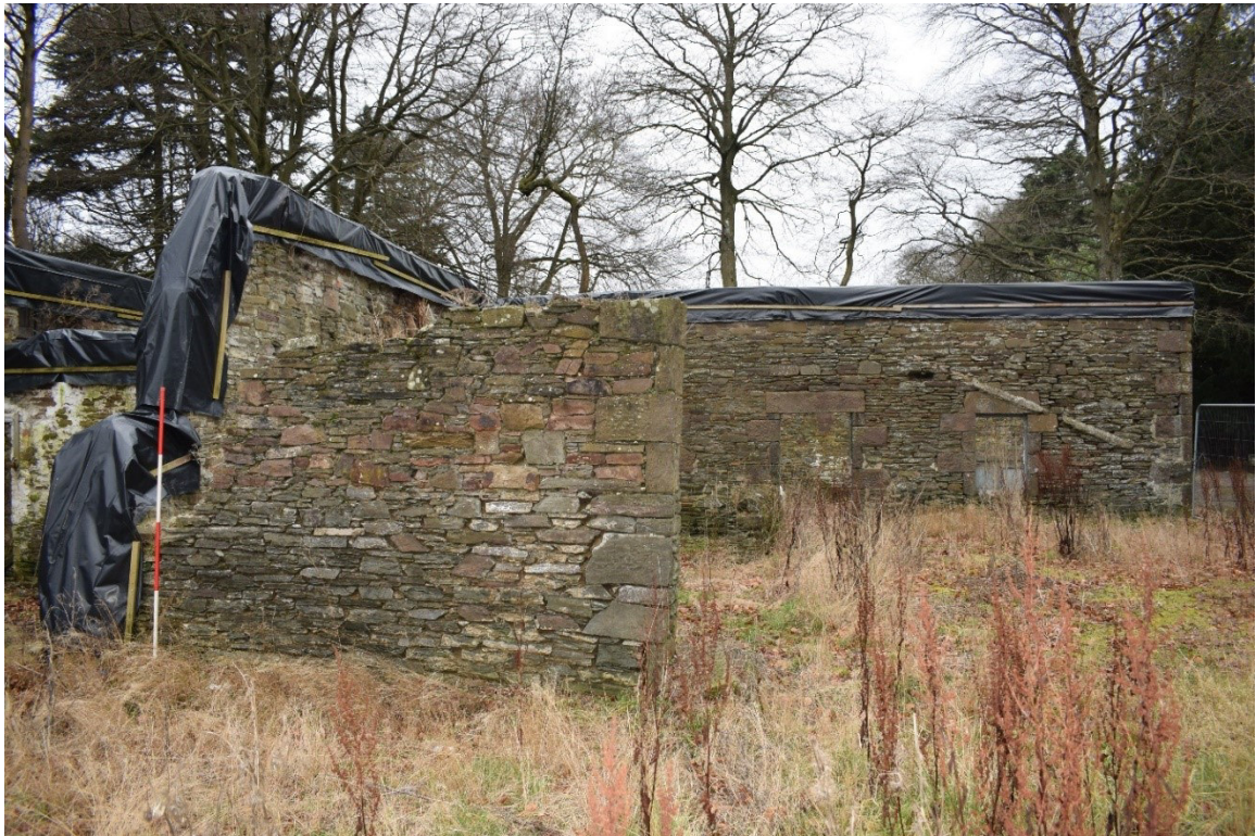
Illus 9 Wall F27 (left) showing lower (earlier) half grey sandstone and upper half with quoins and red sandstone rubble; facing WSW
