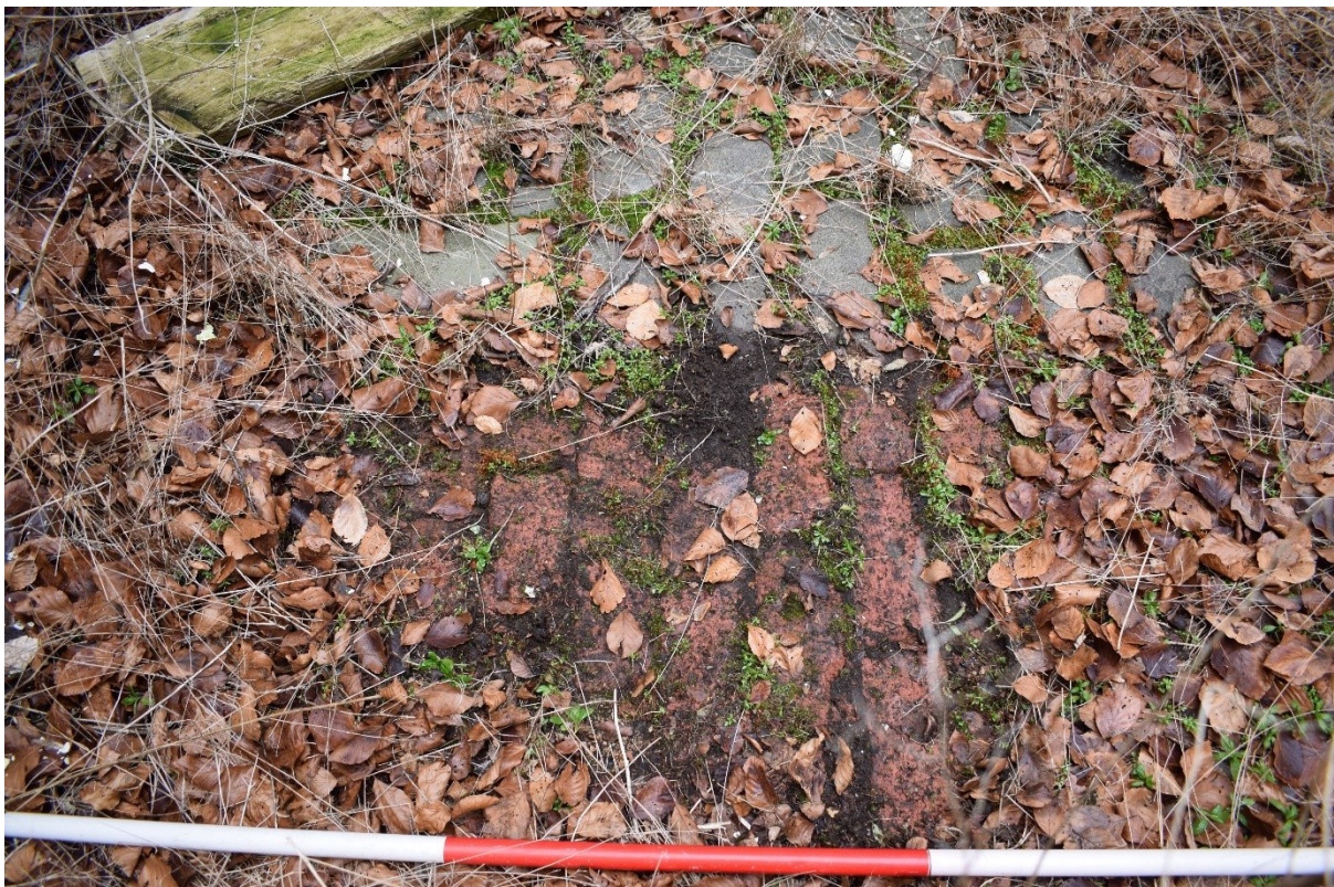
Illus 26 Room 2 former stables floor F9 granite cobbles (top) and hand-made bricks (bottom); facing ENE
