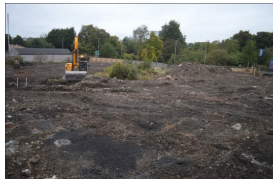
Plate 1: Pre excavation area from south-west
