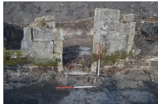
Plate 3: Detail of door in room B from south
