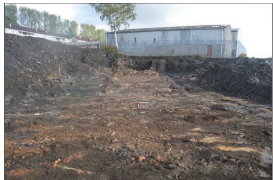
Plate 7: Post excavation of building 003 from west
