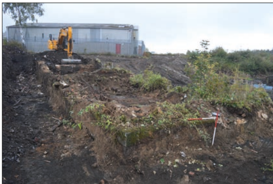
Plate 2: General view of building 003 from north-west
