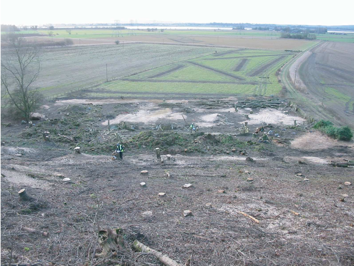
UFC05-GLT: Plate 1 - General shot, before clearance (facing S)
