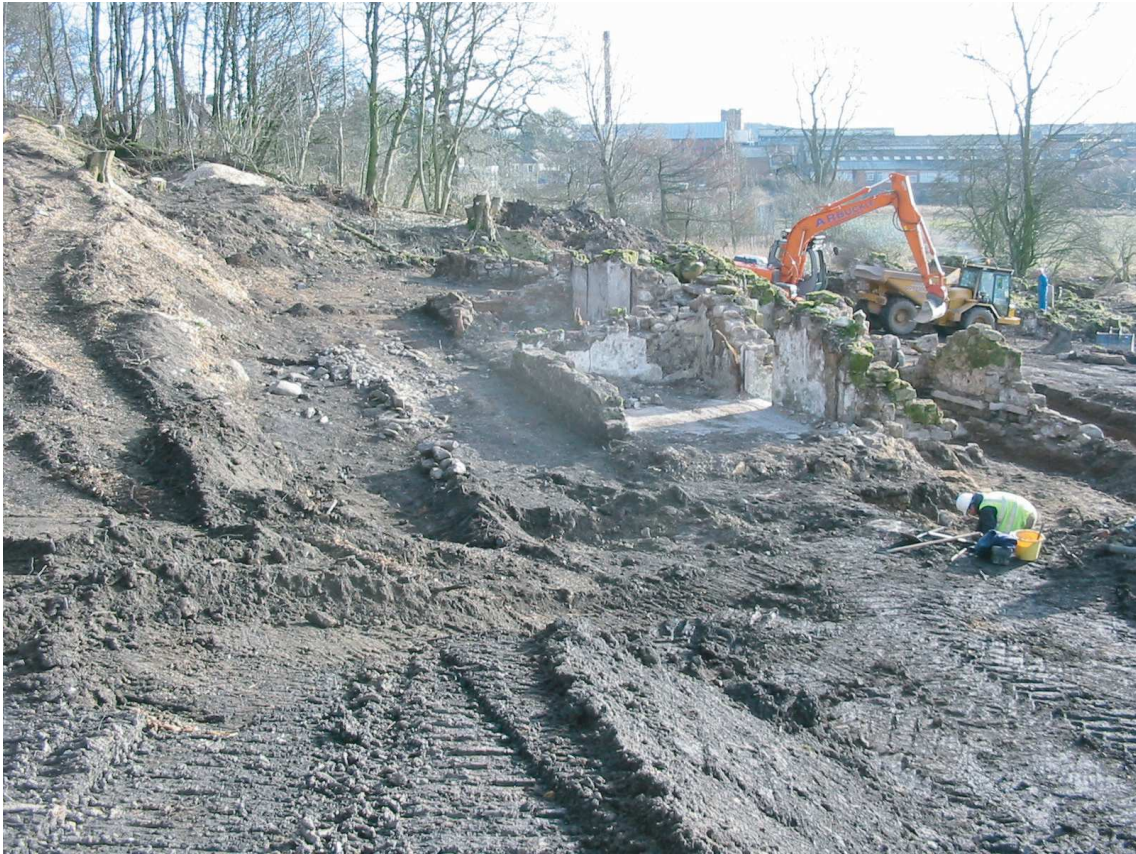
UFC05-GLT: Plate 3 - Rear of house showing surfaces and track (facing E)
