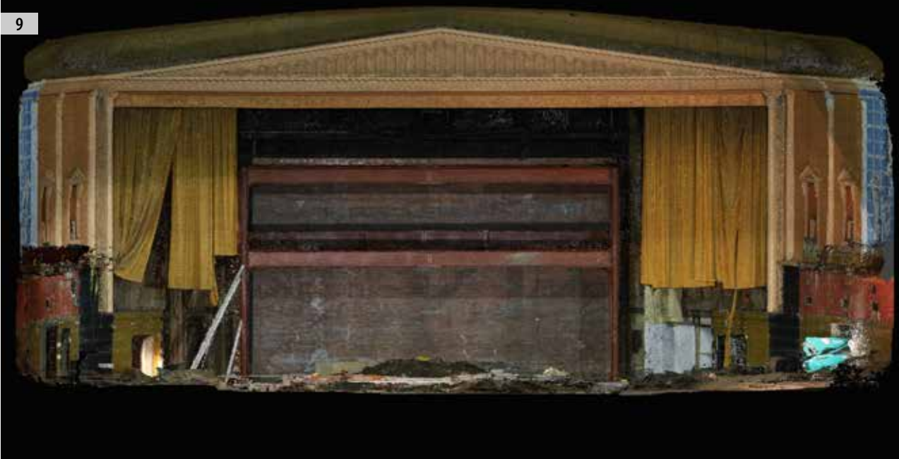
ILLUS 8 Ortho-image of crush hall ceiling, clearly showing restored plasterwork in white. This gives a great idea of the scale of the space in the original cinema ILLUS 9 View of photogrammetric 3D model of west elevation of auditorium.
