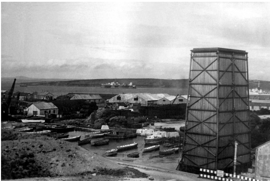
Plate 1 - Cooling tower and surrounding buildings, showing its close proximity to the Pump House to the right (Lindsay & Dobney 2014. Image: The National Archives, ref. ADM116/5790)
