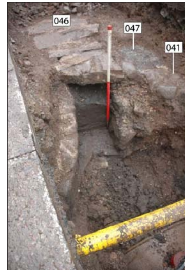
Plate 17: Culvert 046 and mortar and cobbled surfaces 047 and 041, from the north-east
