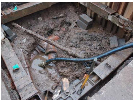
Plate 15: Manhole 3 showing disturbance by numerous services, from the south.
