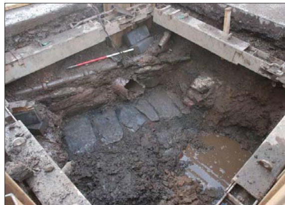
Plate 16: Culvert 035 in manhole 3 from the north-west
