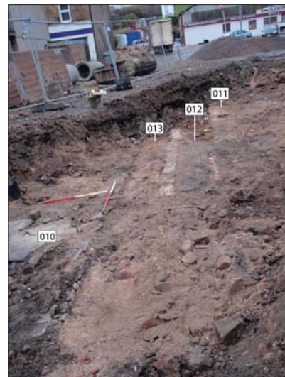
Plate 9: Building remains associated with the demolished Kinloch Distillery
