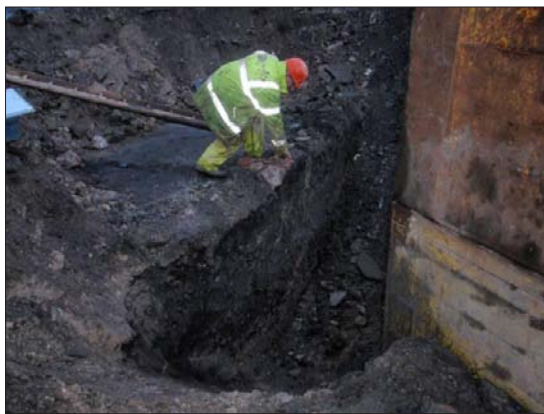
Plate 8: Wall [009] and concrete floor (010), from the south-east
