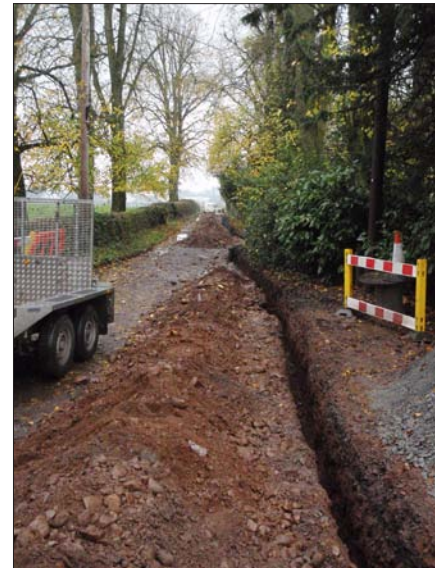
Plate 1- general view of excavated trench from north-west end.
