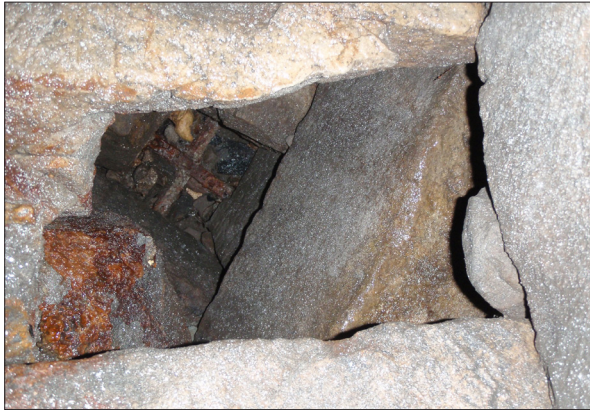
Plate 1: Side drain entering main drain at roof height identified by RCAHMS.
