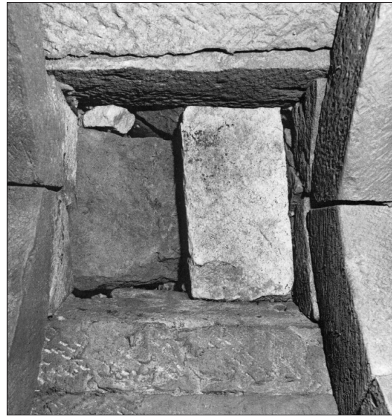
Plate 2: Possible medieval manhole in roof of main drain identified by RCAHMS.
