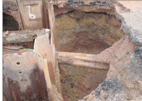
Plate 2: Working shot – piles, frame and fibre optic cables
