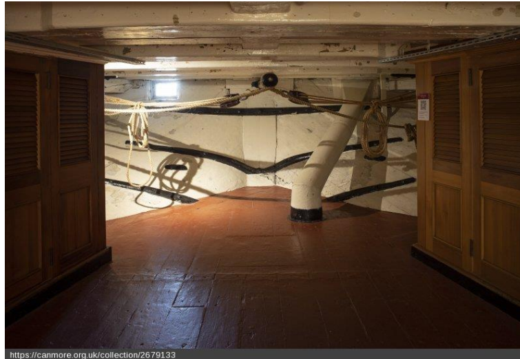
Lower Deck, astern. View of diagonal bracings, internal stern post and tiller rope system (DP 416385, HES, 2023)
