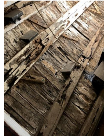
Hold. Hull showing copper fixings reducing effects of salt water corrosion (M.McDonald, 2023)
