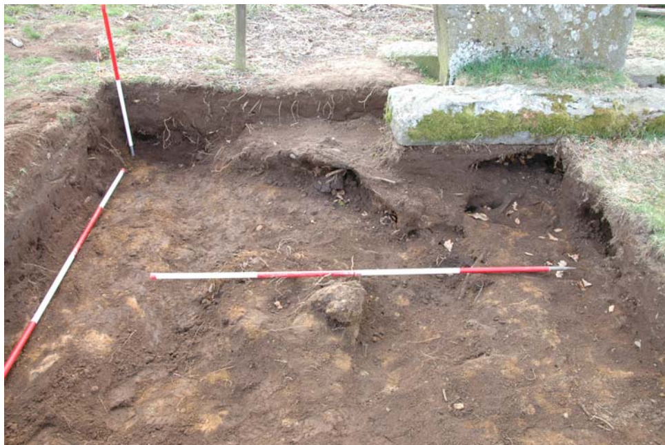
Illus 10 Trench to natural in foreground. Context 3 visible at back. Furrow to LHS.
